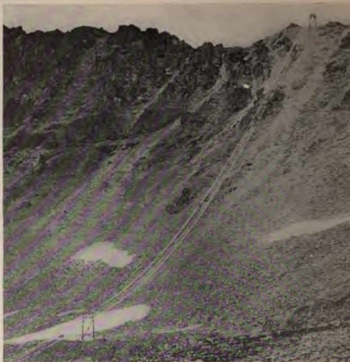
FIG. 4.—LONG SPAN AT CAMP BIRD DIVIDE.
